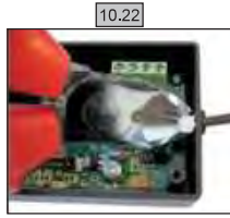
10.22 Cut the flange.
