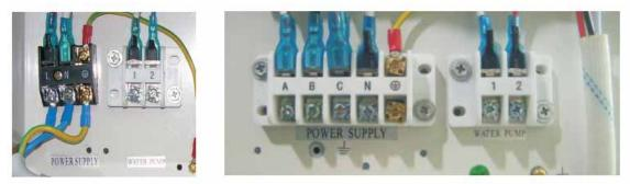
**Remarks**: for models with 3 phases, switching 2 phases may cause an inversion of the rotational direction of the electrical motors, which could damage the unit. Therefore, a protection device has been built in, which will interrupt the circuit if the connection has not been carried out correctly.
